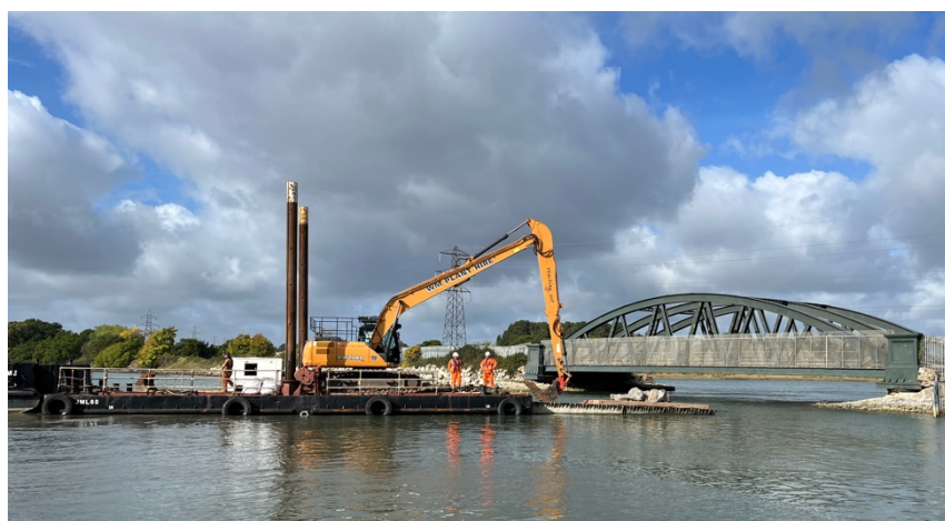
Figure 1: One of the excavators on the barge approaching the viaduct
